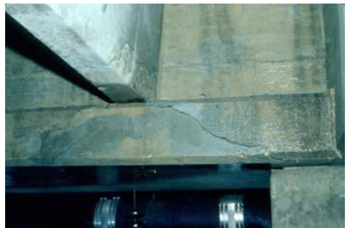
Fig. 1: A typical form of ledge distress
