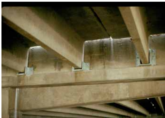
Fig. 2: Added steel support brackets under tee stems
