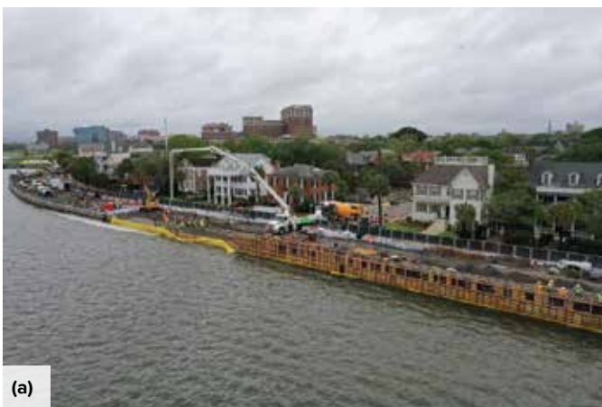
Fig. 3: Phase II of the concrete seawall project: (a) a straight section of concrete placement; and (b) placed concrete and installed GFRP reinforcement in the straight seawall section
