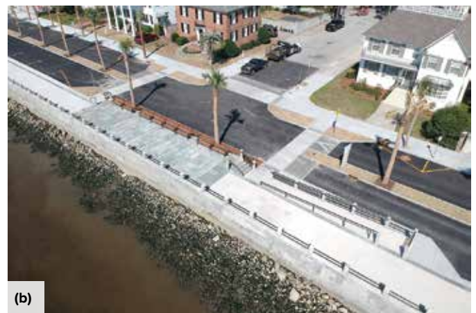
Fig. 3: Phase II of the concrete seawall project: (a) a straight section of concrete placement; and (b) placed concrete and installed GFRP reinforcement in the straight seawall section
