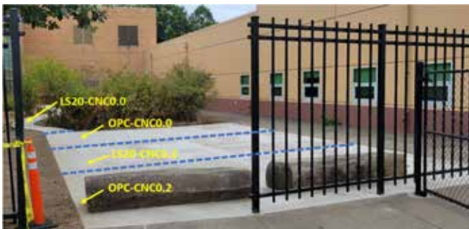
Fig. 5: The site after placing the slabs and the walkway
