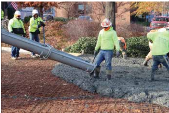
Fig. 2: The 0.2% CNC mixture being placed for the parking lot
