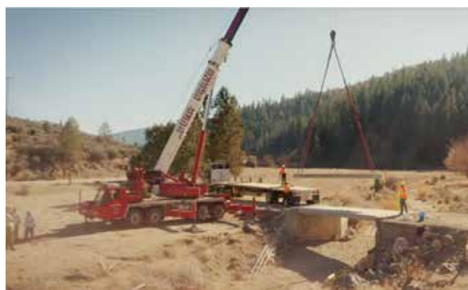
Fig. 4: Placement of the box girders
