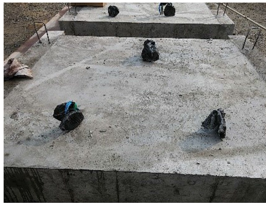
(i) Cast-in-place (CIP) overlay concrete casting
