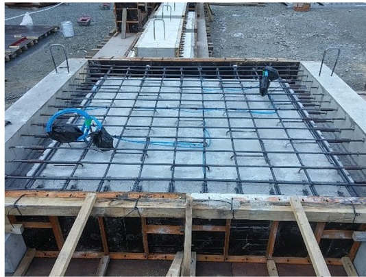
(h) Upper rebar assembly
