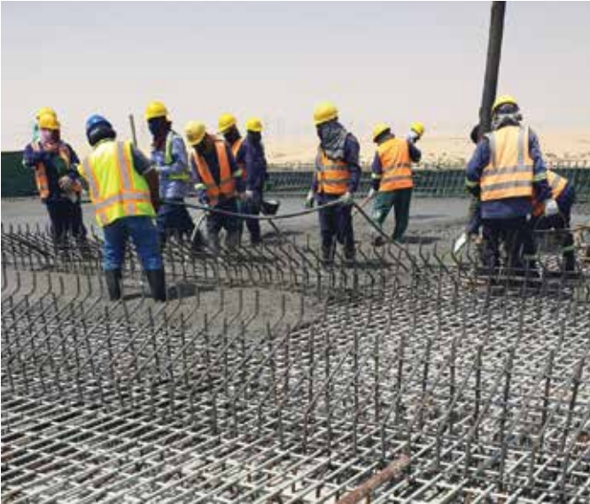
Fig. 6: GFRP bar installation and concrete placement at the SPARK bridge
