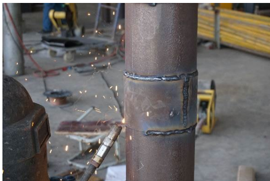
(e) Overall welding of steel strip
