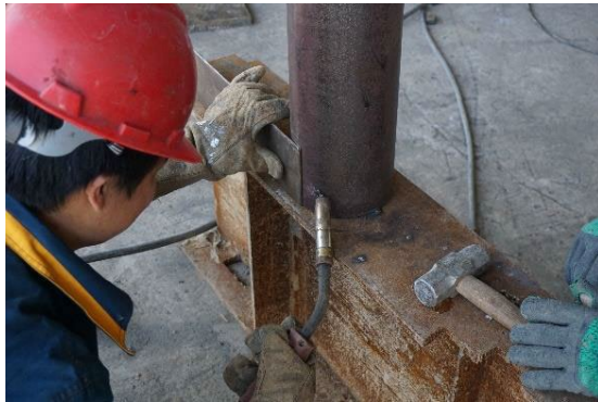
(a) Weld one end of the steel strip
