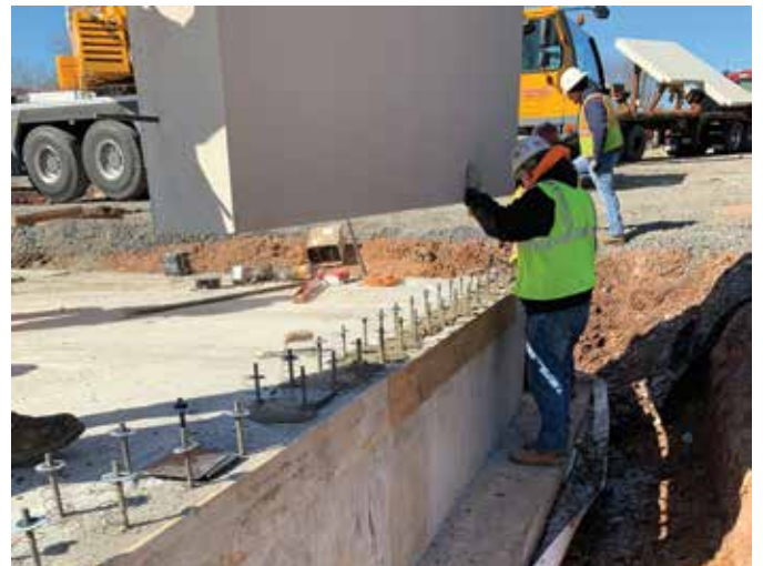
Fig. 6: Prefabricated panel installed over reinforcing bars cast into the foundation
