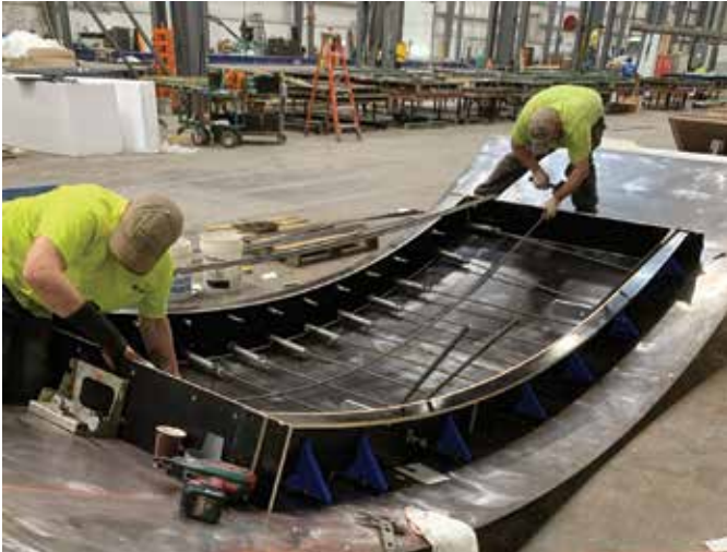
Fig. 5: Installation of reinforcement grids in a curved panel (left) and the panel after casting (right)
