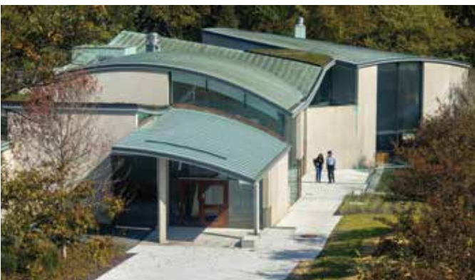
Fig. 3: Roof with varying curving levels
