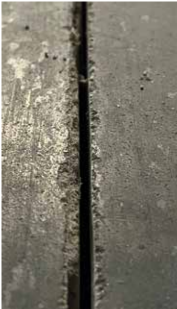
Fig. 9: Saw cutting too early results in raveled joint edges (photo courtesy of Scott Metzger, Metzger/McGuire)
