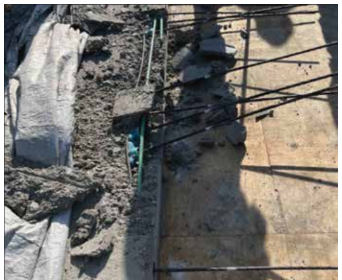
Fig. 12: Tendons in a concrete slab constructed with Type IL concrete were stressed based on a maturity calibration for Type I cement concrete. The strength of the Type IL cement concrete was overestimated, resulting in slab blowouts
