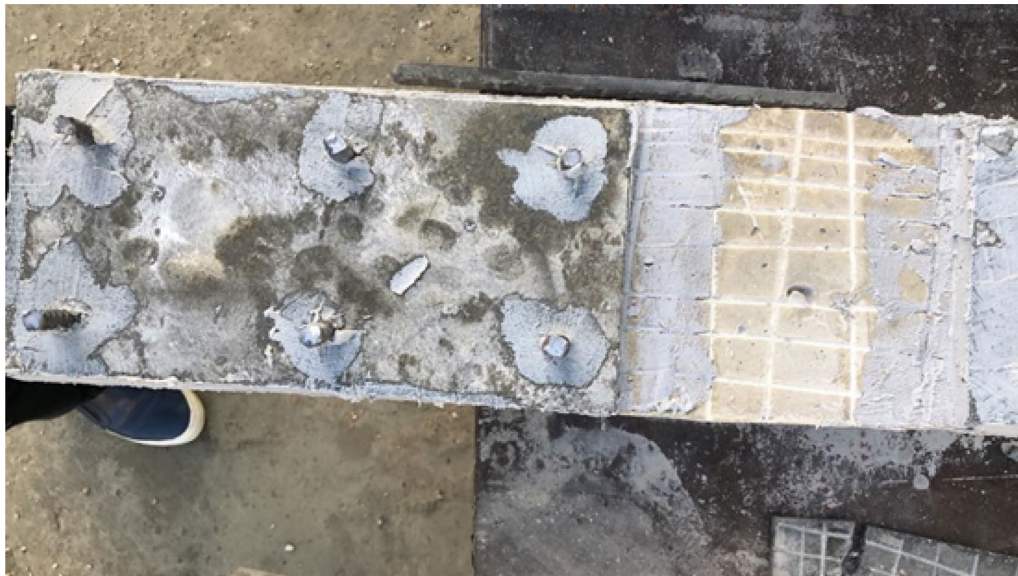
Fig. 7 Strengthening scheme with HPFRC plates
