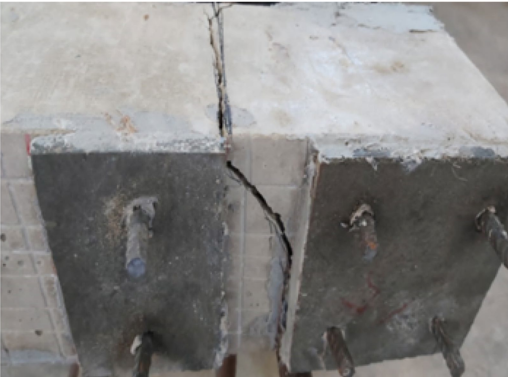
Fig. 12 RC beam without stirrups strengthened with vertical HPFRC strips
