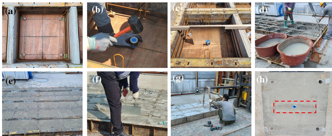
Fig. 8 Fabrication process of cracked concrete blocks
