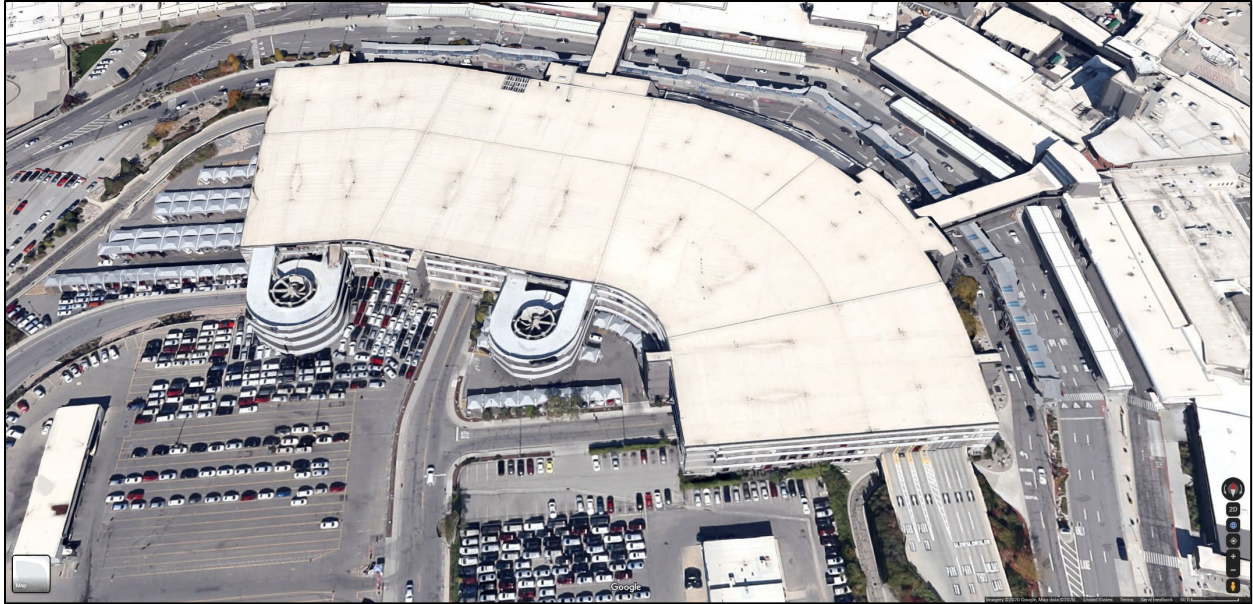
Figure 1-2 3D rendering looking north onto the parking garage, obtained from Google Maps, image from 2020 before demolition began.
