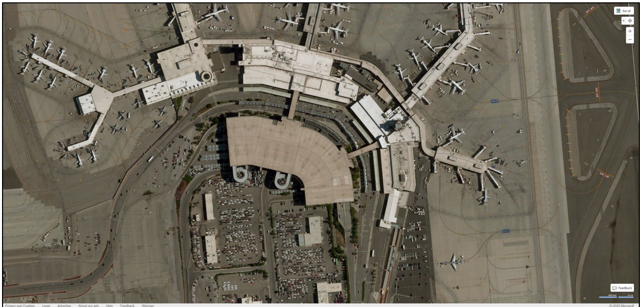
Figure 1-1 Aerial photograph of the SLC airport and parking garage obtained from Bing.com, image from 2020 before demolition began.
