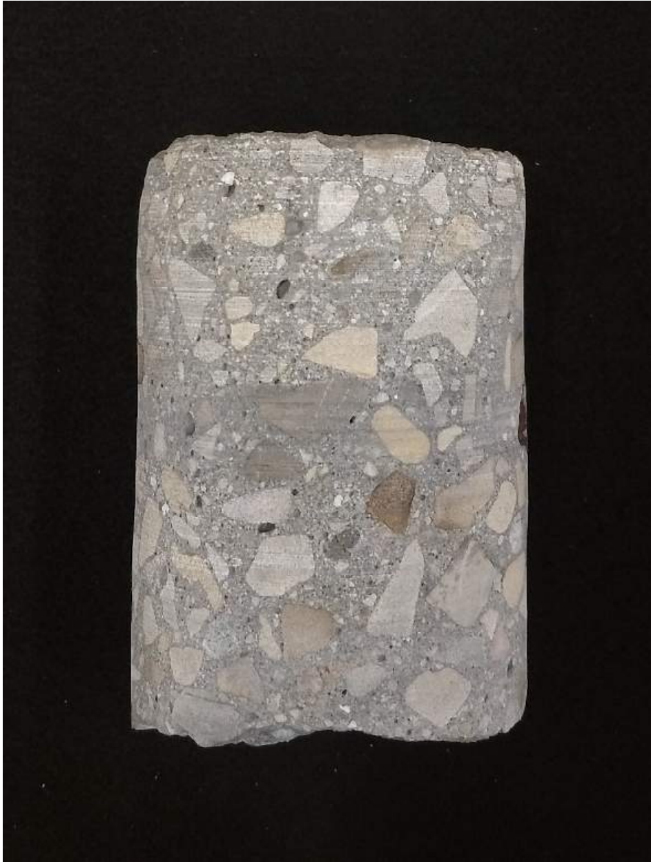
Figure A-7: Core Lane 4
