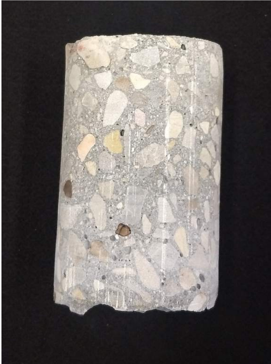
Figure A-6: Core Lane 3
