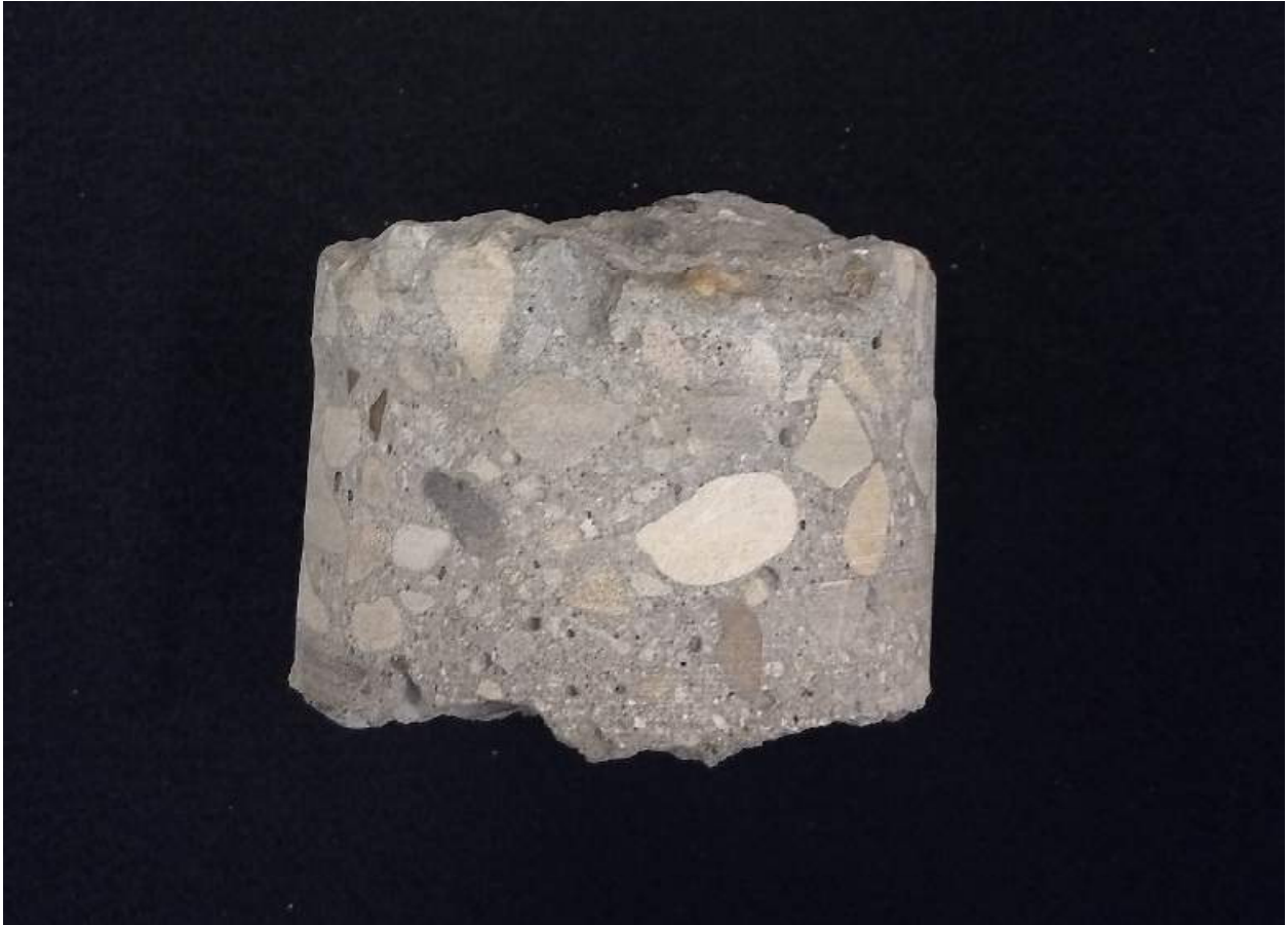
Figure A-10: Core Lane 6 (Bottom)
