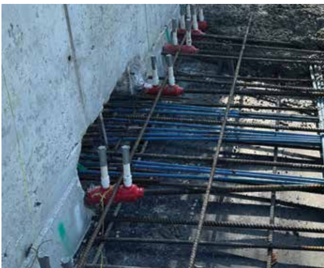
Fig. 4: PS=Ø slab-to-wall restraint relief joint
