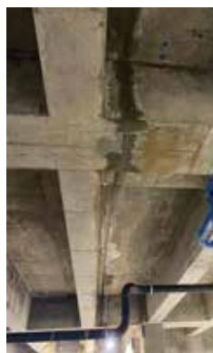
Fig. 7: PS=Ø beam-to-beam restraint relief joint
