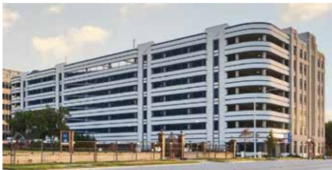
Fig. 8: Hospital parking garage in Texas with PS=Ø technology
