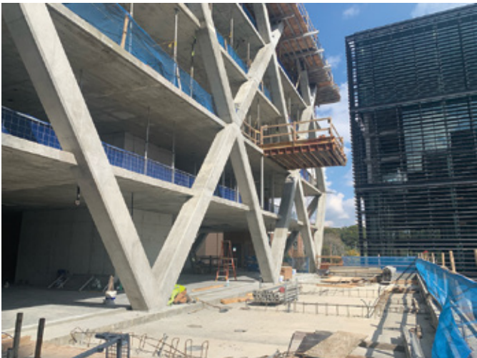
Fig. 2: View of the façade showing the columns sitting 12 in. (305 mm) proud of the slab
