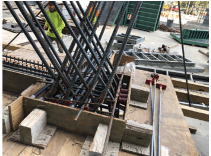
Fig. 4: Reinforcement mockup of the corner column/slab joint
