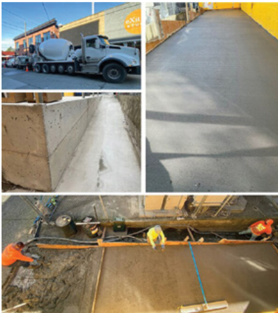
Placement of C-Crete's basalt-based concrete
