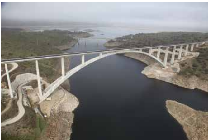
Viaduct Over River Almonte, Garrovillas de Alconétar, Cáceres
