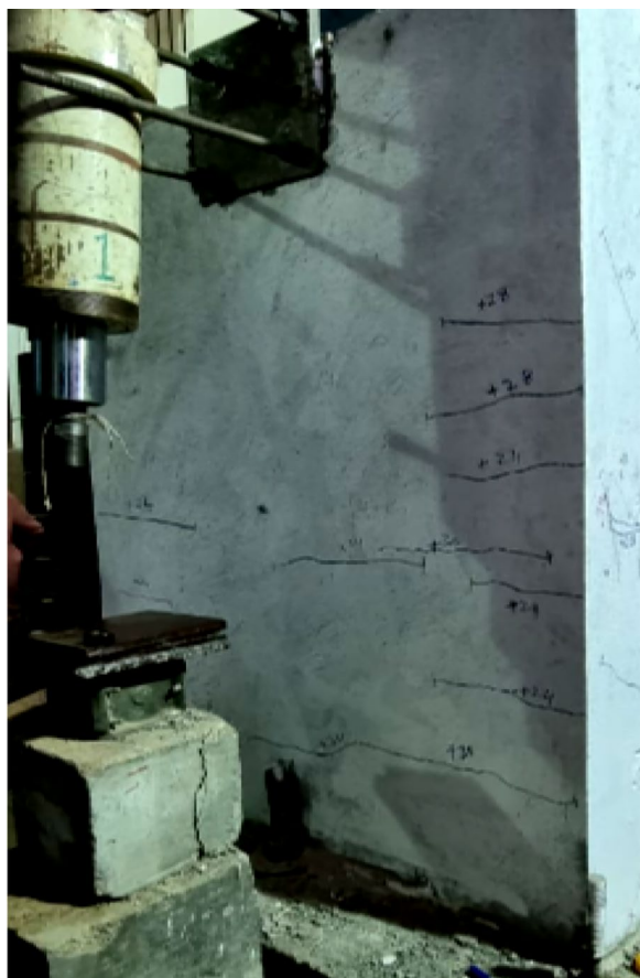
Fig. 19 Failure crack pattern S-02 (left)
