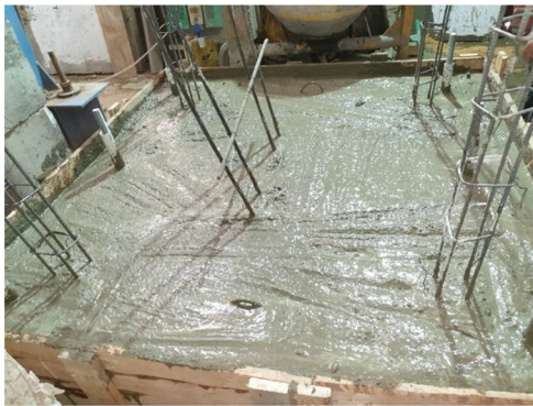
(a) Base footing and columns dowels
