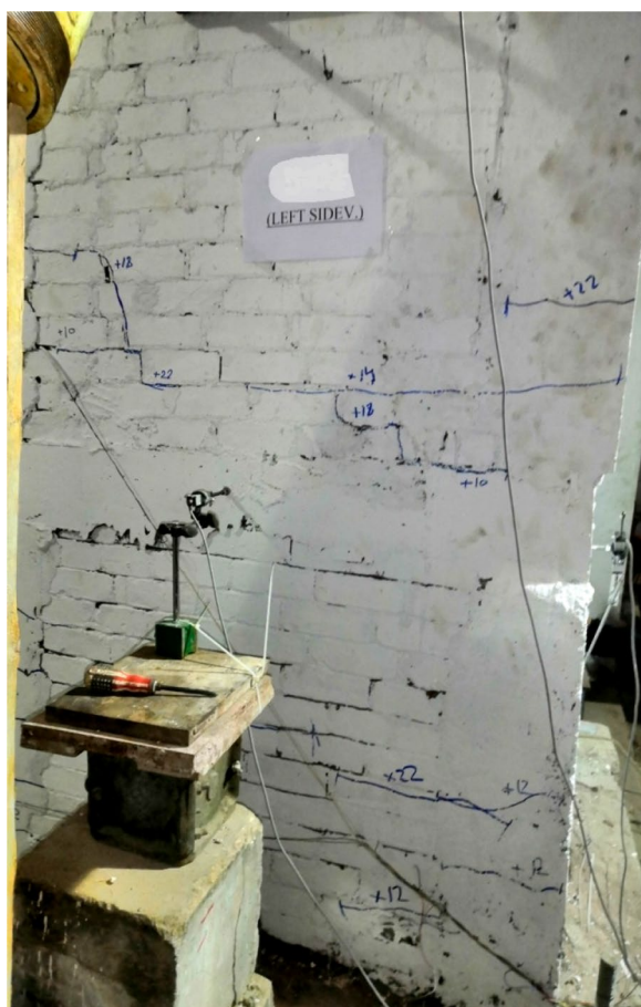
Fig. 13 Crack failure pattern S-01 (right)
