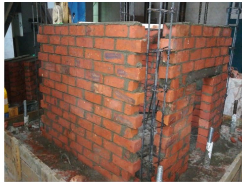
(b) construction of level 1 masonry walls
