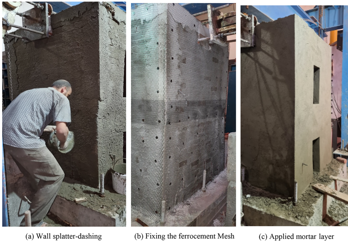
Fig. 4 Ferrocement’s retrofitting 3D assembly procedures
