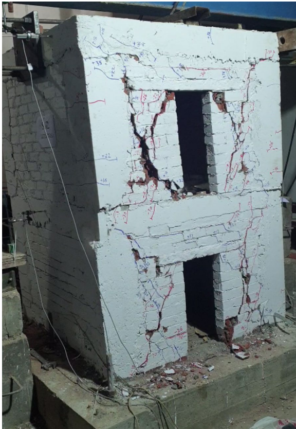
Fig. 11 Crack failure pattern S-01 (back)
