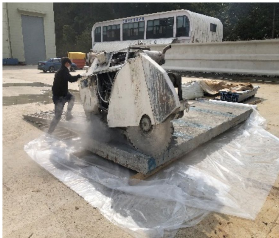
Fig. 1 Concrete deck remolding
