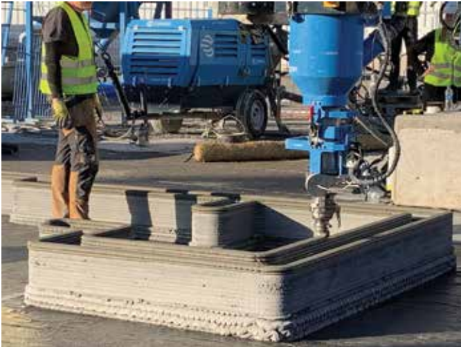
A 3-D-printing demonstration at World of Concrete, Las Vegas, NV, USA
