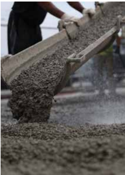
Fiber-reinforced concrete placement
