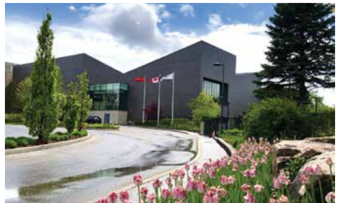
The Granite Club Garage Rehabilitation Project
