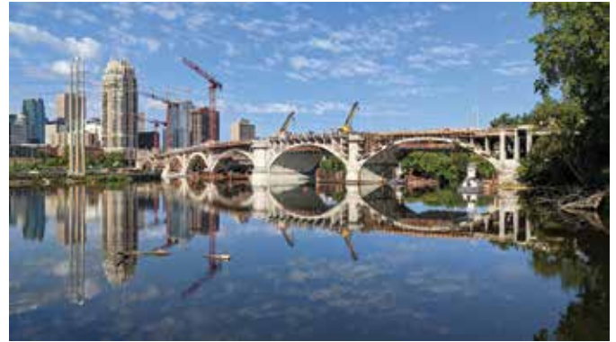
View of historic 3rd Avenue Bridge during rehabilitation
