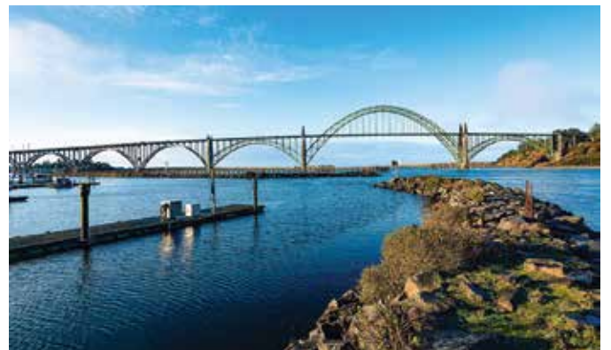
Yaquina Bay Bridge Cathodic Protection Rehabilitation
