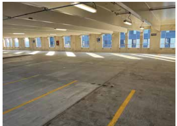
NEIU parking deck after repairs
