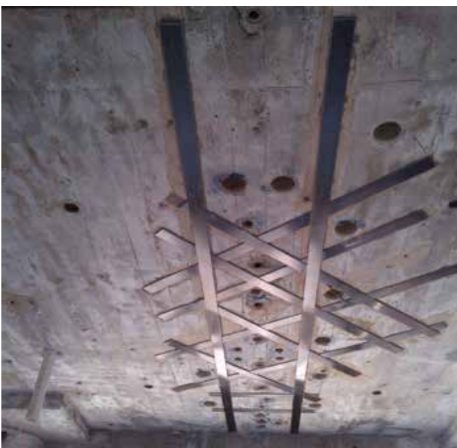
Carbon fiber plates were installed for strengthening
