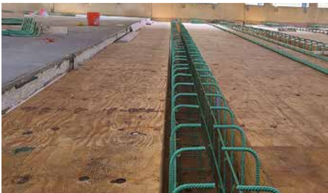
Partial reinforcing bar detail with formed repair
